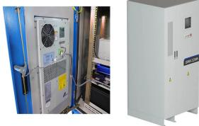
How do energy storage systems work? Energy Storage Systems are structured in two main parts. The power conversion system (PCS) handles AC/DC and DC/AC conversion, with energy flowing into the batteries to charge them or being converted from the battery storage into AC power and fed into the grid. Suitable power device solutions depend on the voltages supported and the power flowing.
